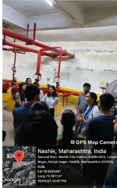
Maintenance team explaining how the Fire safety protocol are followed
