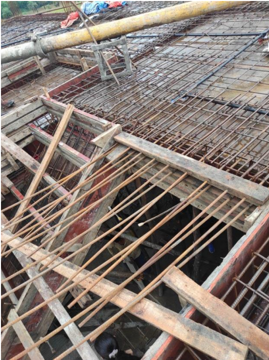
Reinforcement casting on site
