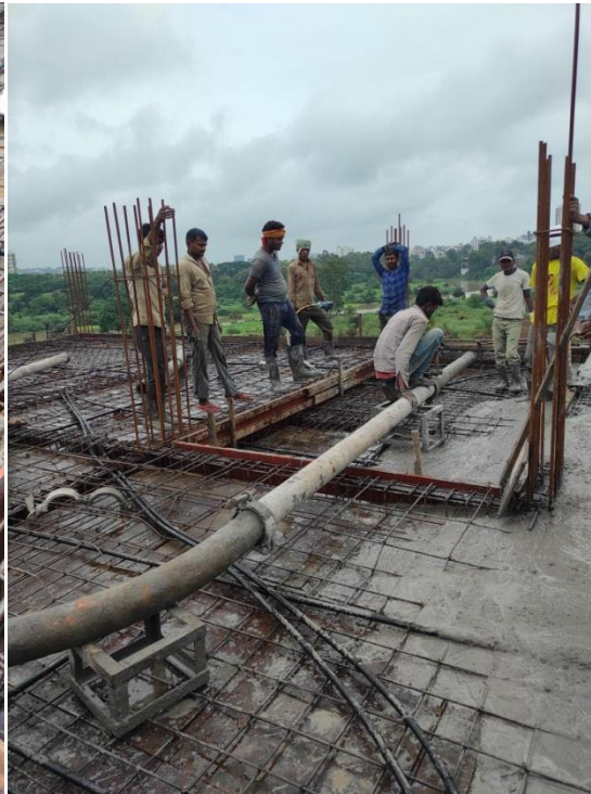
concrete pouring on site
